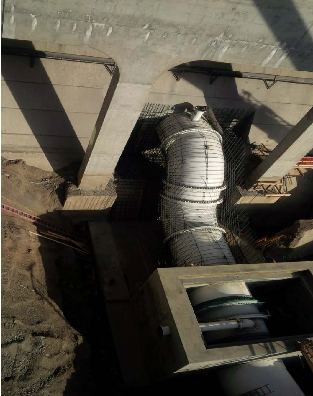
Rebar forming for concrete encapsulation upstream of 10' valve room.
